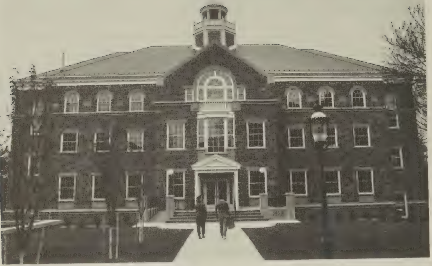
Templeton Hall — Completed 1989
